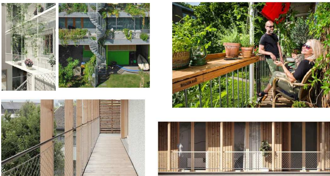
materialisering borstwering appartementencomplex
