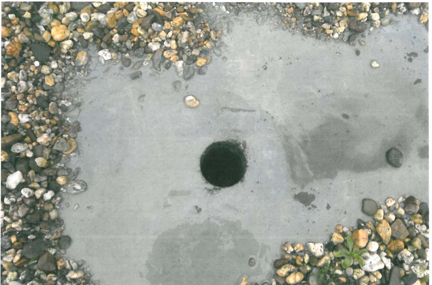
BOZ 10092 - Westhavendijk 14-16 Middelharnis (boorgat 3)
