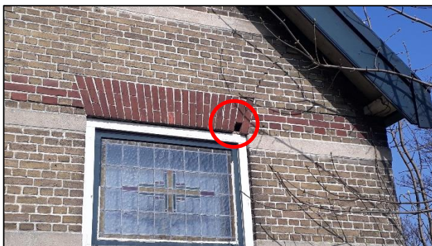
Foto 5: Opening in muur
