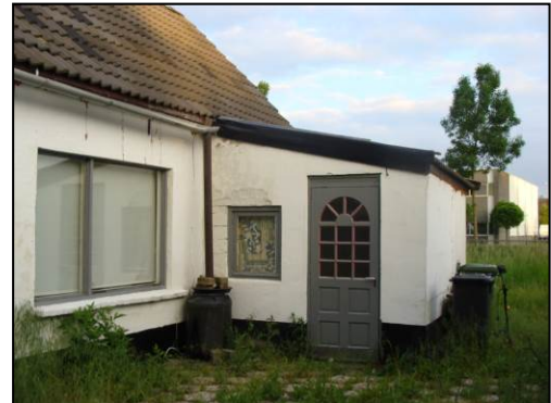
Foto 2. Te slopen woning
