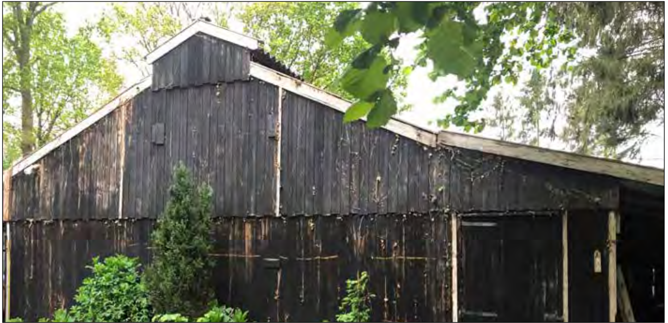
te slopen kippenstal
