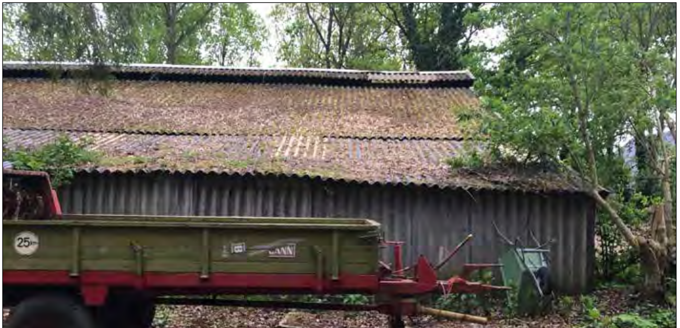
te slopen kippenstal
