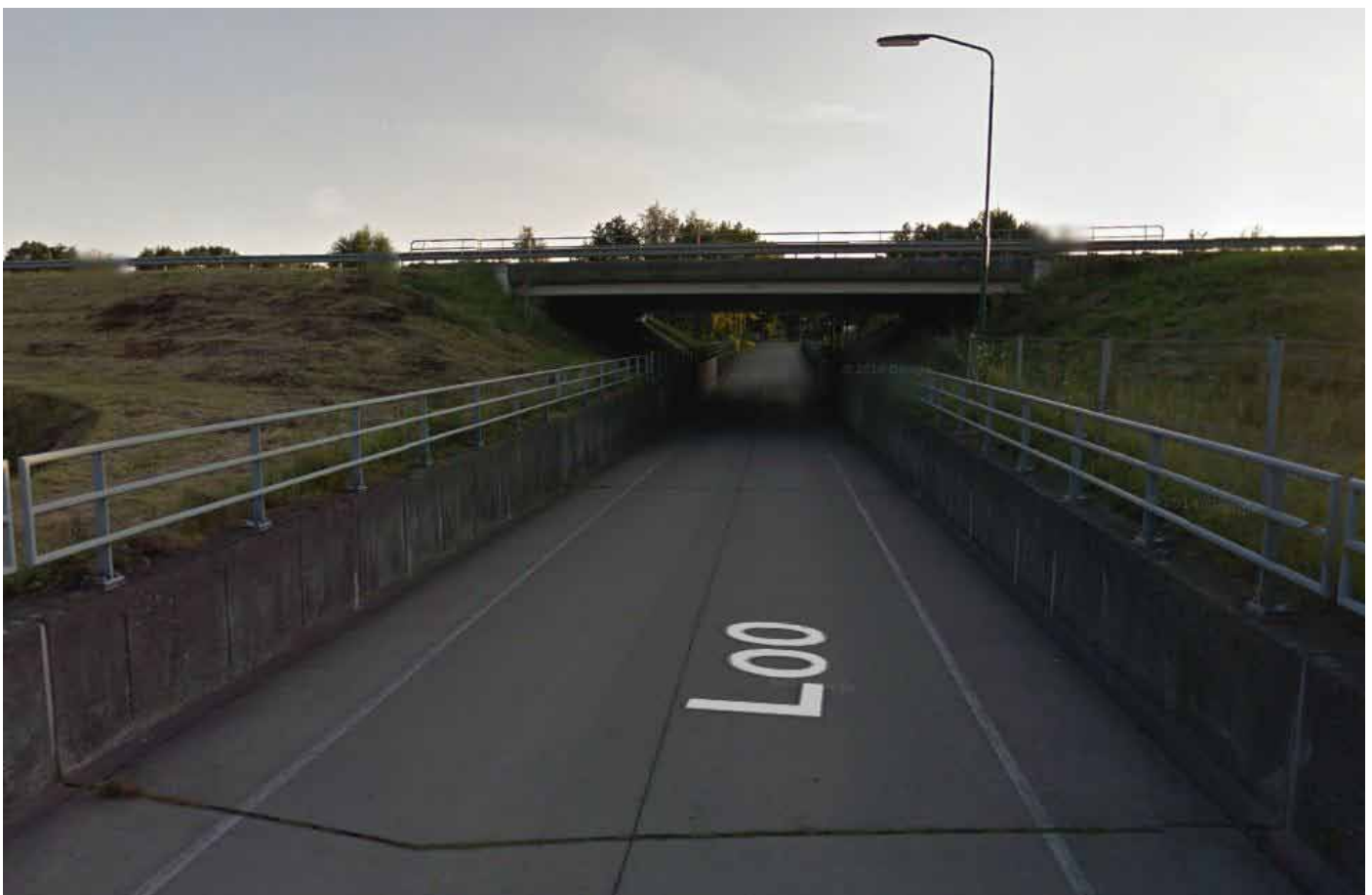
Tunnel onder A50 (bron: Google streetview)
