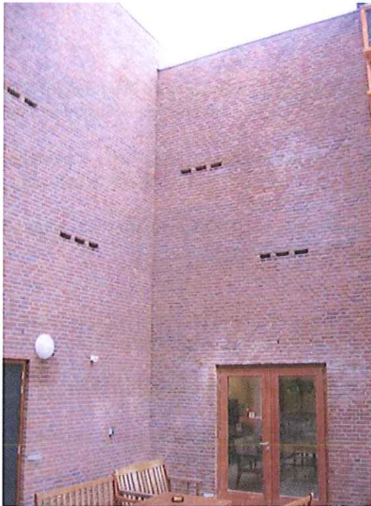
Foto 22: Spouwkasten in kantoor WNF in Zeist
