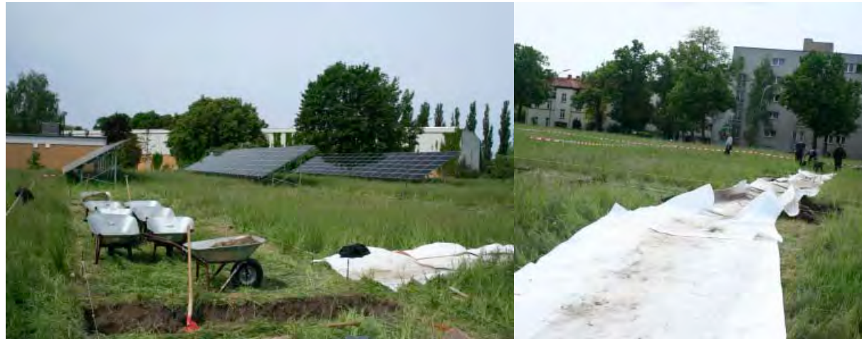
Wheelbarrows were used to remove excavated earth during the building work on the Tegel waterworks site. Because of the high ecological value of the sites, protected plants were transplanted and geo fleece was used to minimize trampling damage (right). (Photo: Tim Peschel)
