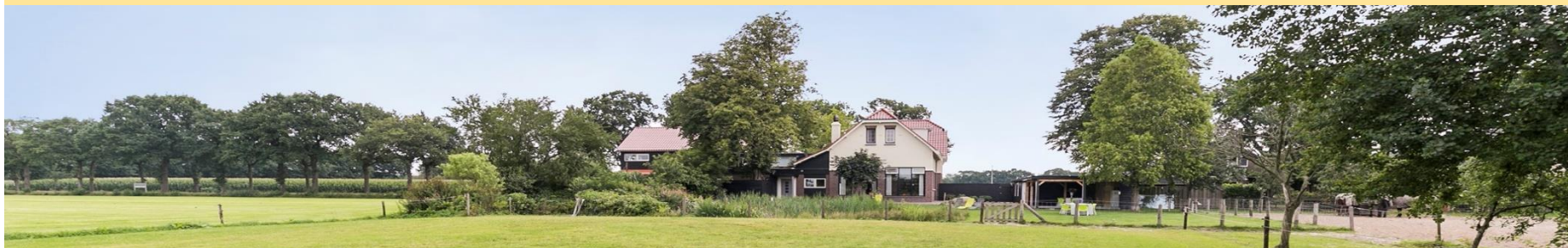
Herbestemming Lagere school Wateren 22 december 2021
