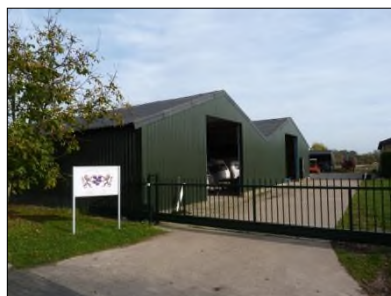
Figuur 8. Loods / caravanstalling.
