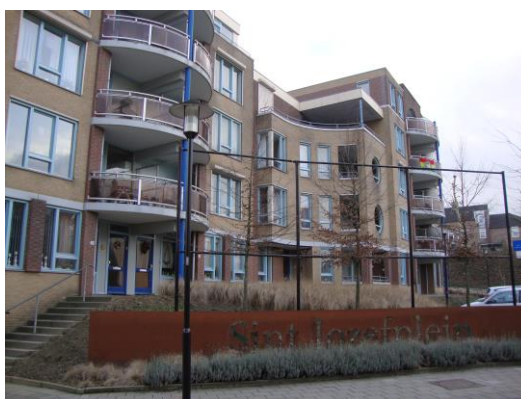
Appartementencomplex St. Jozefplein
