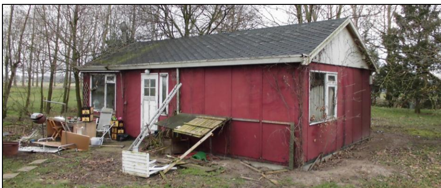
Te slopen woning
