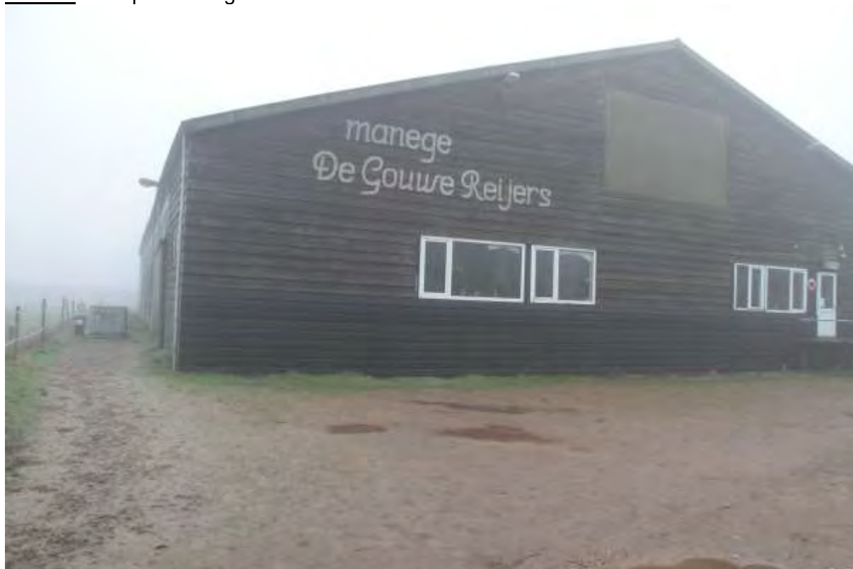
Foto 1. Te slopen manege.
