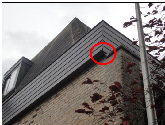
Foto 1. Openingen in dakrand hotel
