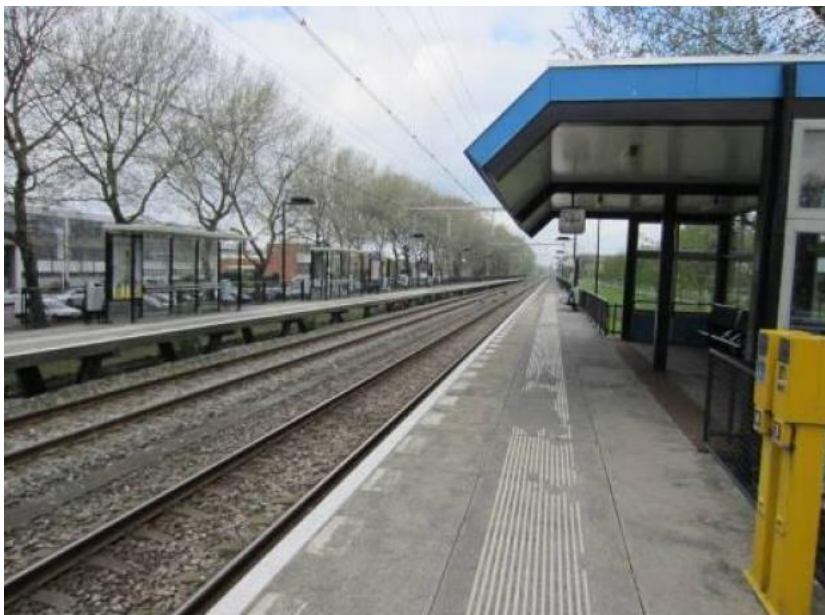
Figuur 3 Station Vlaardingen West
