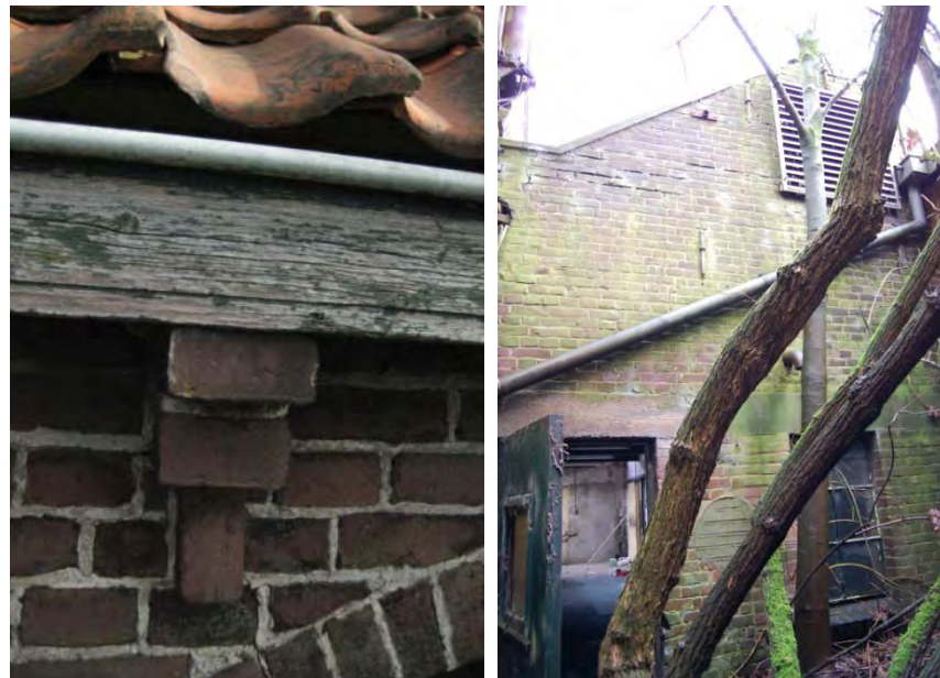
Links: gemetselde console in de westgevel
