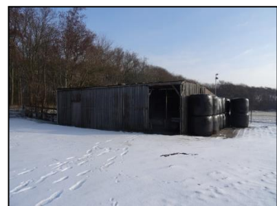
Figuur 5. Te slopen loods.
