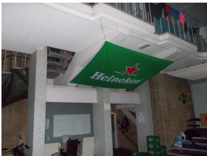
Detail betonnen trap hal
