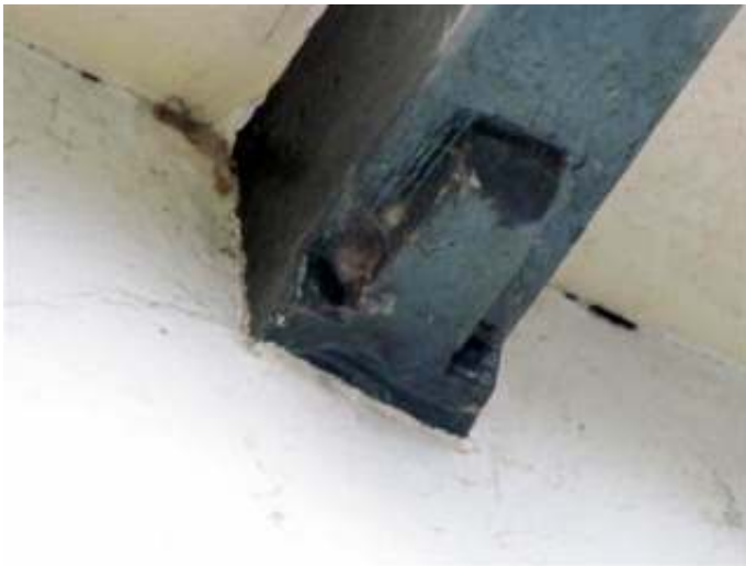
Figuur 10: gedichte opening in balk.
