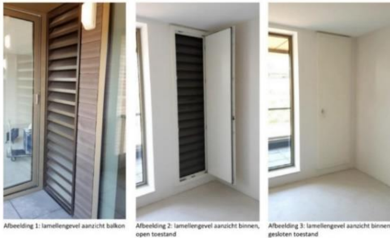
Figuur 10c: Principe comfortbox (red. tot ca. 15 dB)
