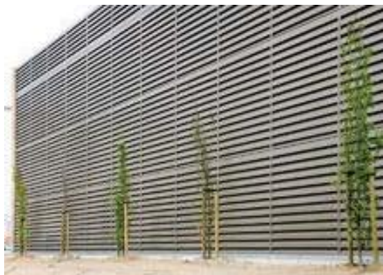
Parkeergarage in Osnabrück (DE)
