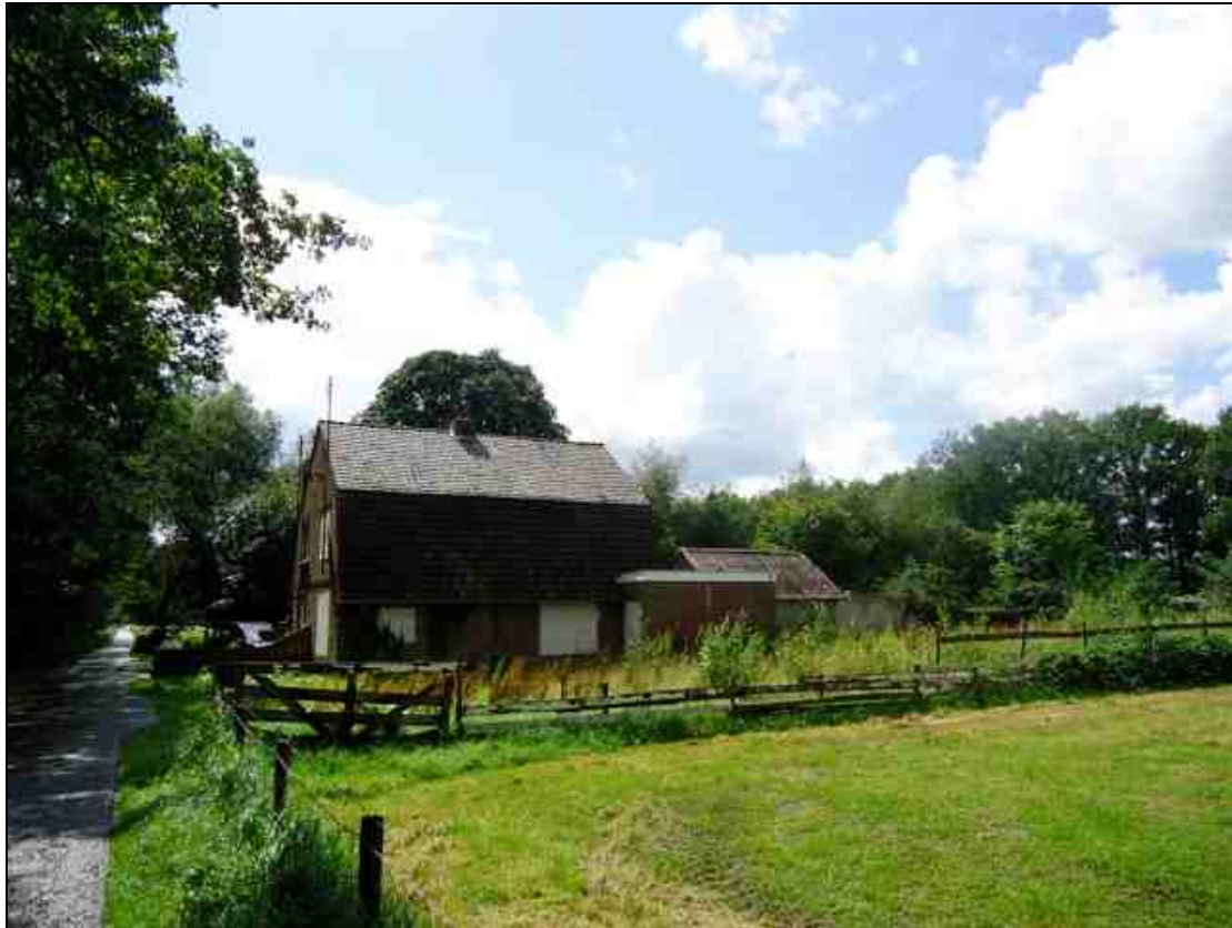
Foto te slopen woning
