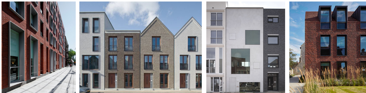
Detaillering is geraffineerd
