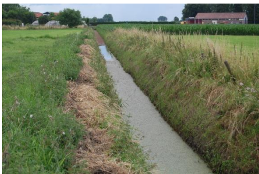
Foto 6 Watergang (noordkant plangebied)
