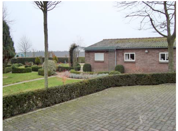
Foto 4. Te slopen woning.
