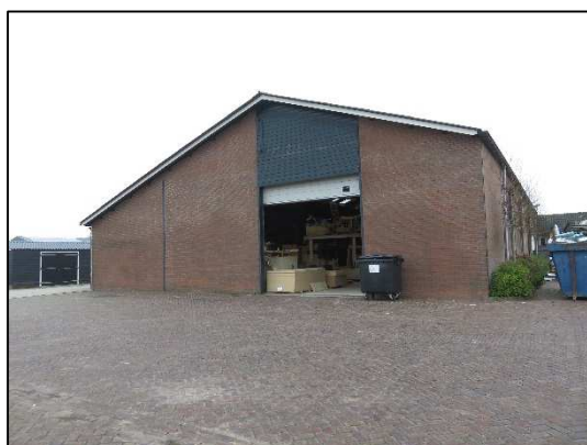
Foto 3 te slopen loods
