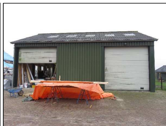
Foto 2 te slopen loods
