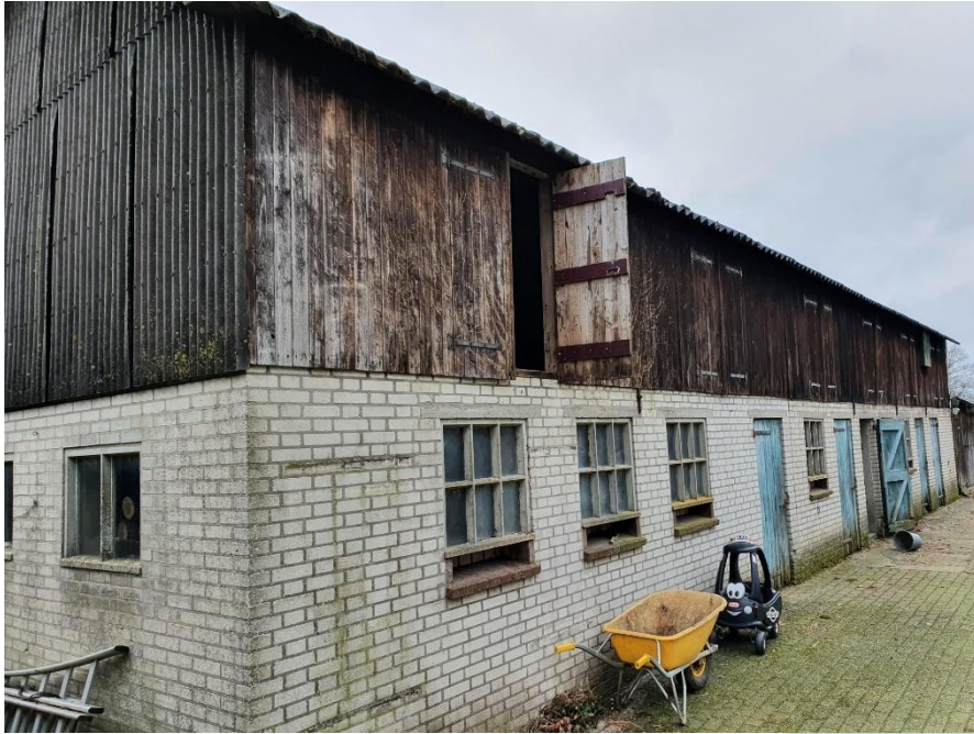
Te slopen stal
