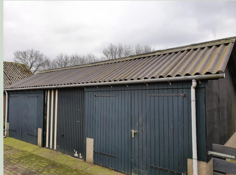
Te slopen garage
