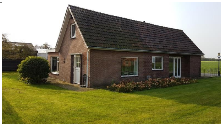
foto 4: te slopen woning
