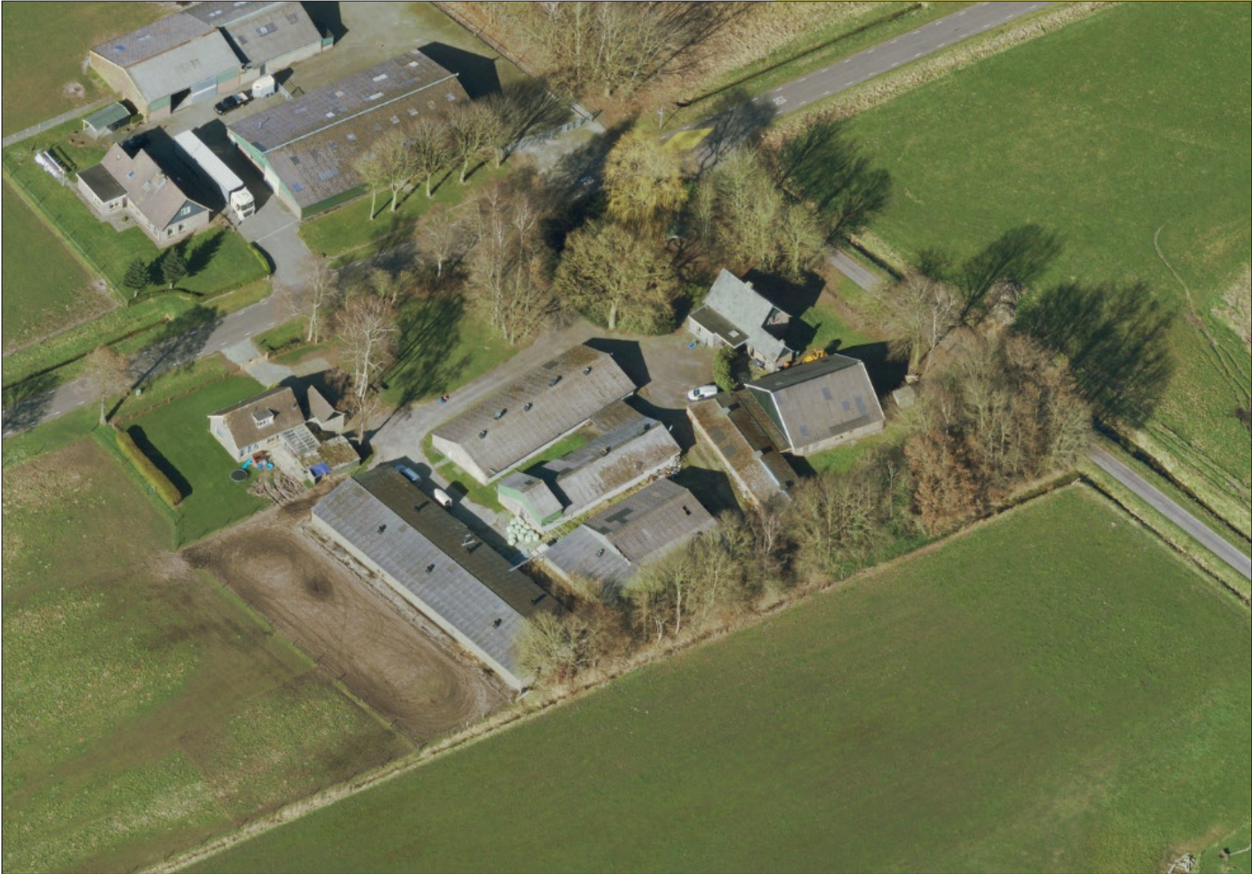
te slopen stallen
