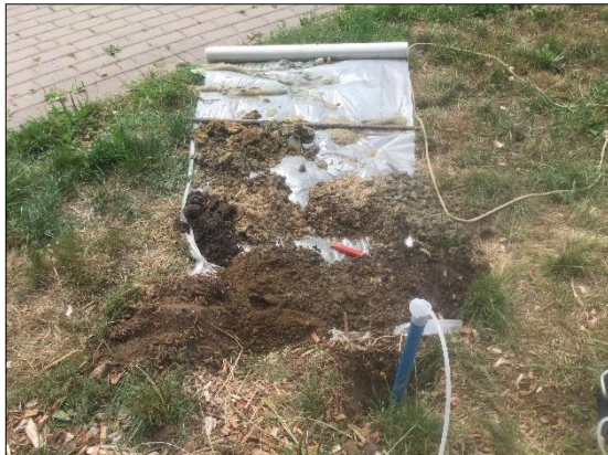
Foto 5: boring 10 (d.d. 17 augustus 2022)
